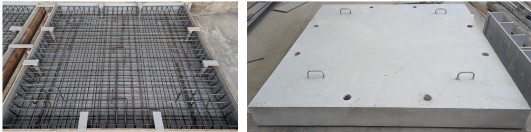
Fig. 2 Reinforcement of the slab S1.2 (left) and concreted slab (right).
