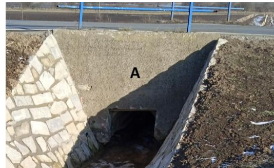
Fig. 2 Photo showing face A of the culvert depicted in Fig. 1 in reality.
