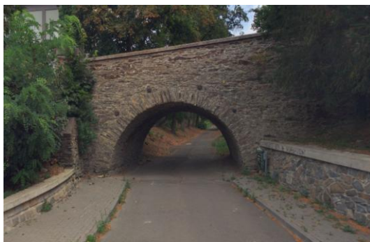
Fig. 8 The surveyed arched stone bridge in reality.
