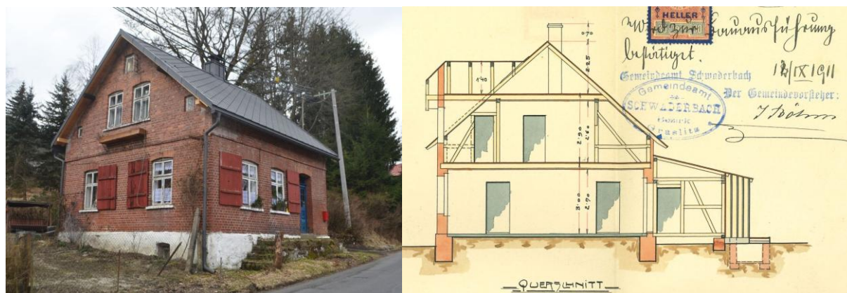
Fig. 1 The view of the case study building in 2024 from the south-east (left). The section of the case study house on the original building plan (right). The house was originally designed without basement and with a dormer which remained unrealised [14].
