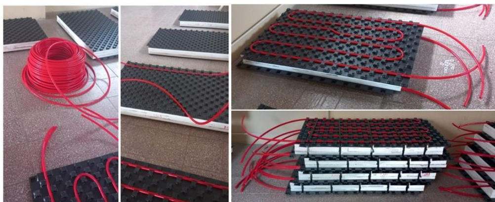
Fig. 5 Piping installation [Author].
