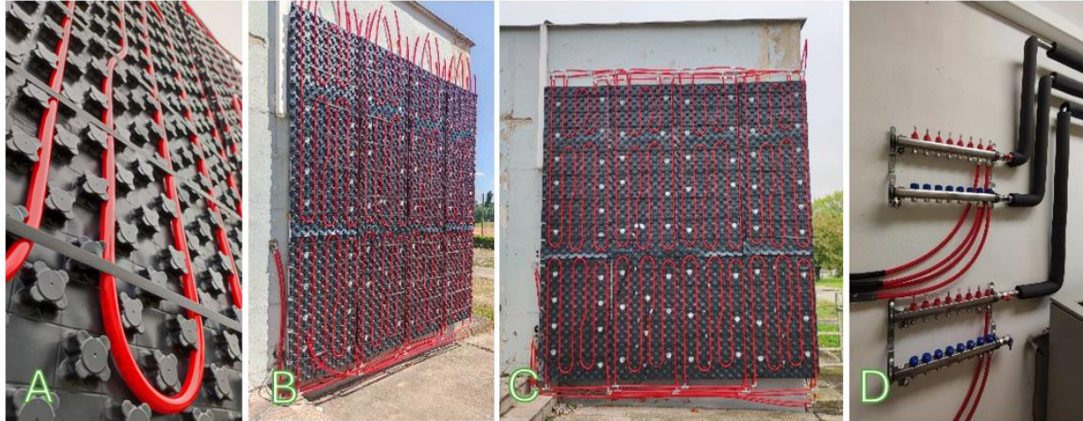
Fig. 8 Finalization of the Building Facade with ATP [Author].
