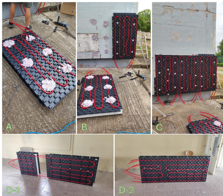
Fig. 7 Application of ATP Panels to the Building Facade [Author].
