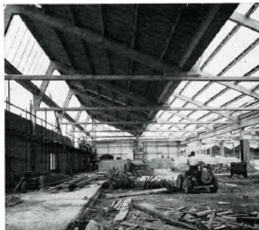
Fig. 17 View of the under-construction roof of the Bristol Workshop Building [13].
