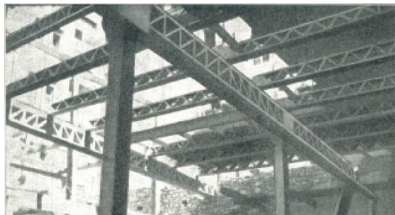
Fig. 6 First concrete truss girders at the beginning of the 20th century [14].
