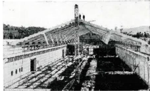
Fig. 19 View of the expanded roof of the Hall in Avilés [13].
