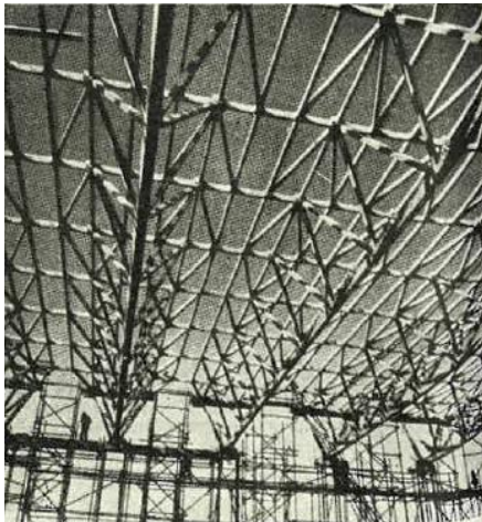
Fig. 13 View of the roof structure under construction at the Gatwick hangar [21].
