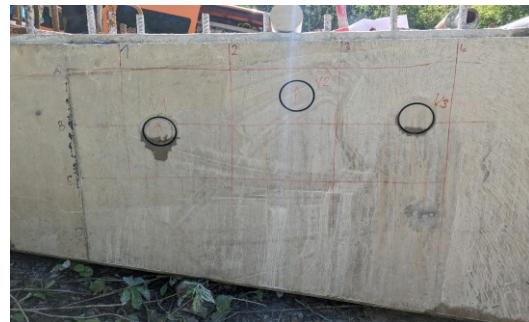
Fig. 2 Core drilling samples from segment A.
