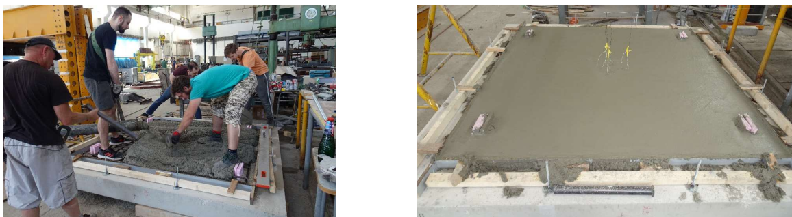
Fig. 7 Casting a layer of concrete overlay.
