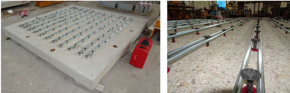
Fig. 5 Injecting shear headed connectors.
