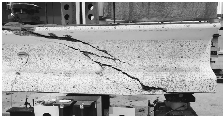
Fig. 5 Beam N 1.1 after collapse.
