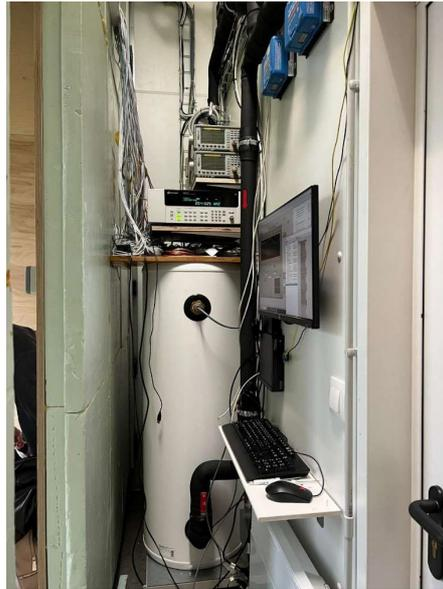
Fig. 4 Compensation space in the Twin Rooms – the space in which the DAQ, a computer with special software and the technical equipment of the experimental facility are located.
