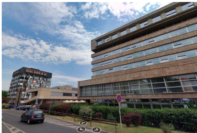
Fig. 2 Building of the Regional Office of the Ústí Region: view from the north, current state. In the left part of the image you can see the insensitively reconstructed facade of the neighbouring originally Brutalist building.
