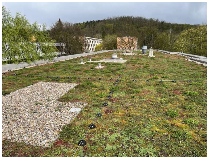
Fig. 1 Green roof in Brno-Komin.
