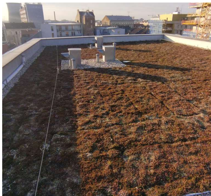
Fig. 2 Green roof in Brno-Bratislavská.
