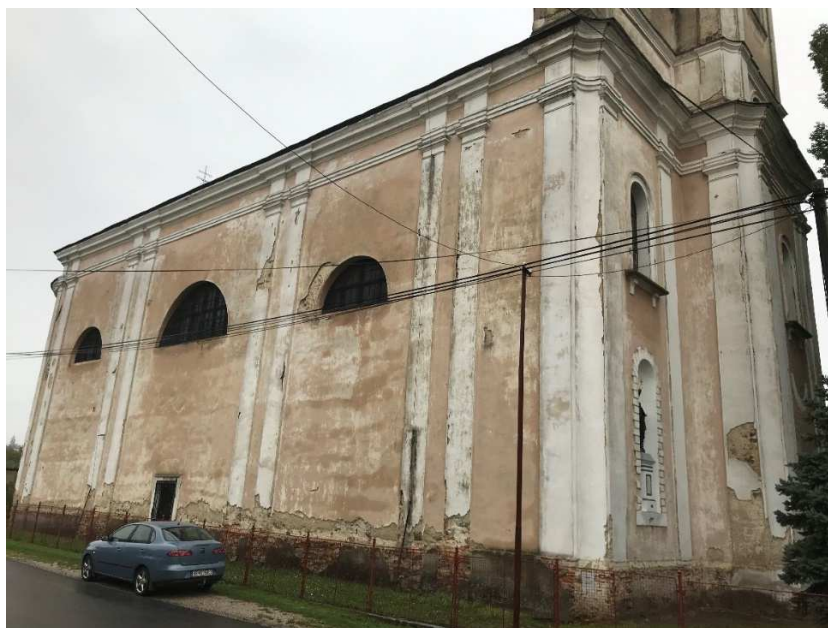
Fig. 1 The actual state of the church's facade (Facade Restoration Project).
