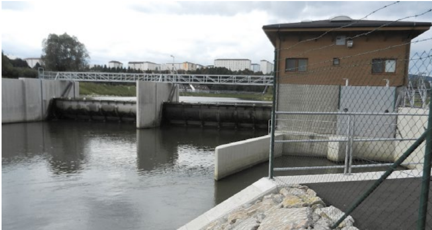
Fig. 1 The small hydropower plant Stará Lubovňa.
