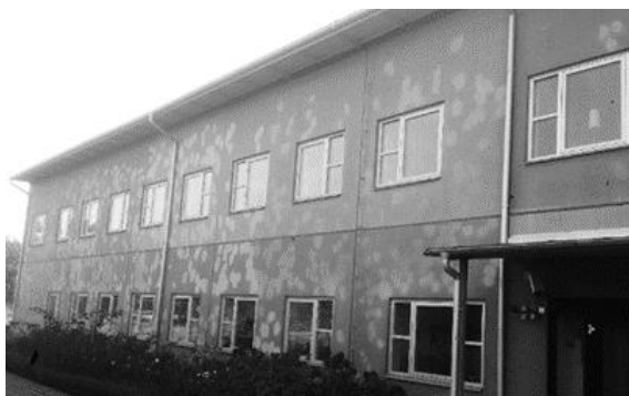
Fig. 1. Facade in Helsingborg during repair.
